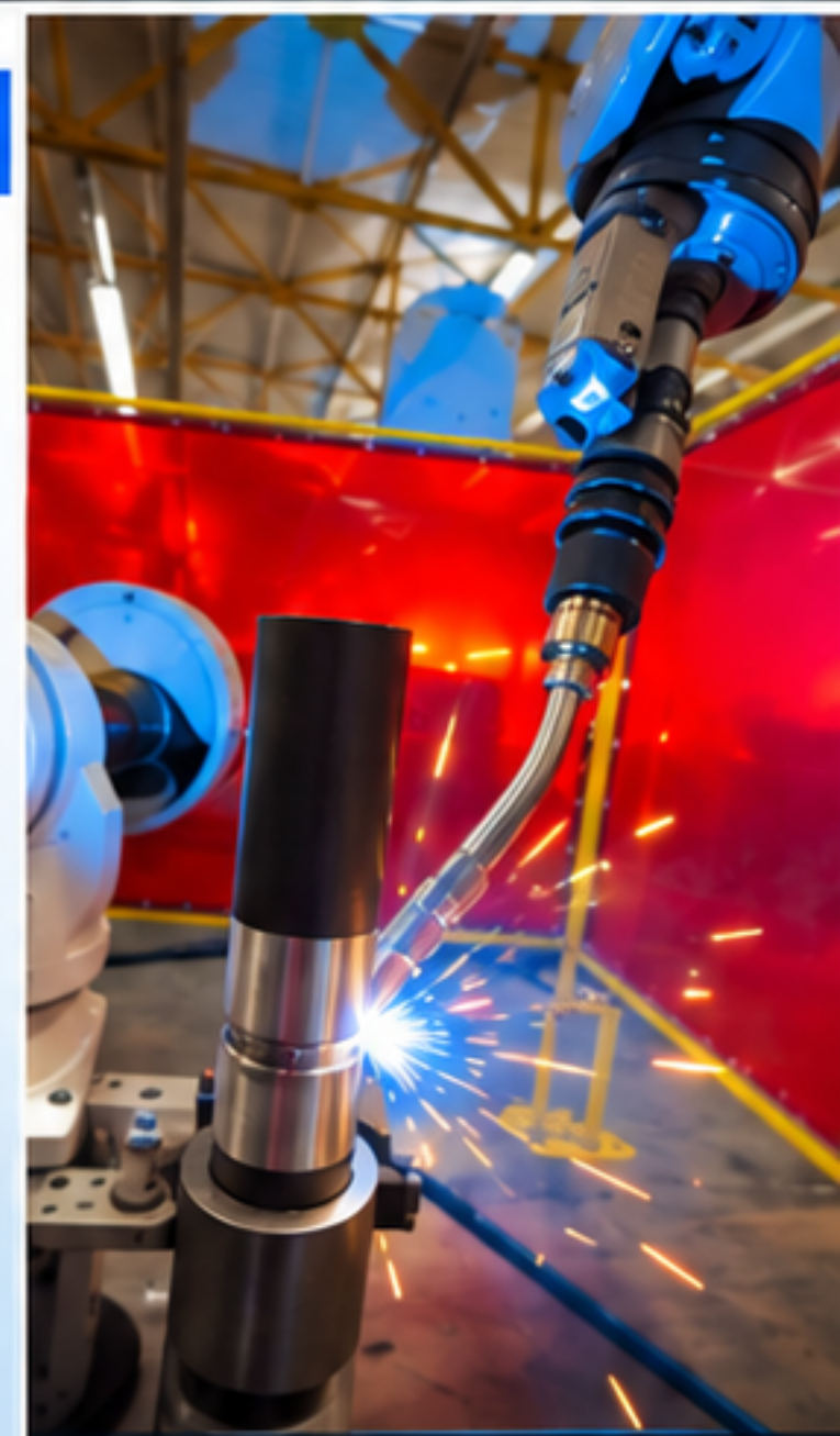
Open Route Pipe Welding
